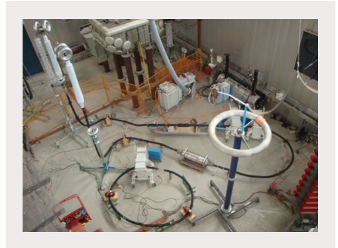
Fig. 16: Type test setup for U_m = 170 kV and 800 mm 2 copper conductor according to IEC 60840
