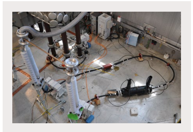
Fig. 11: Setup for the electrical test of the dry type back-to-back joint
