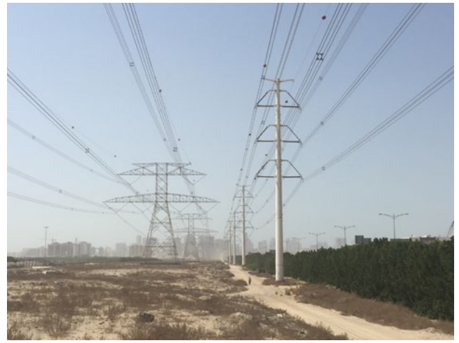
Dubai: Compared with an existing solution (left), this compact line (right) reduces the corridor width by 80 %.
