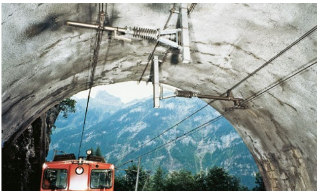
First Railway Line Installation in 1979
