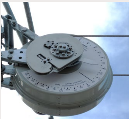
The current operating point can be read off at any time from the scale of the TENSOREX C+.
